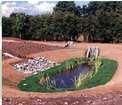
Sustainable drainage systems: Wetland during construction Hopwood Motorway Services Area, Bromsgrove, UK CIRIA SUDS web: www.ciria.org/suds/index.html
